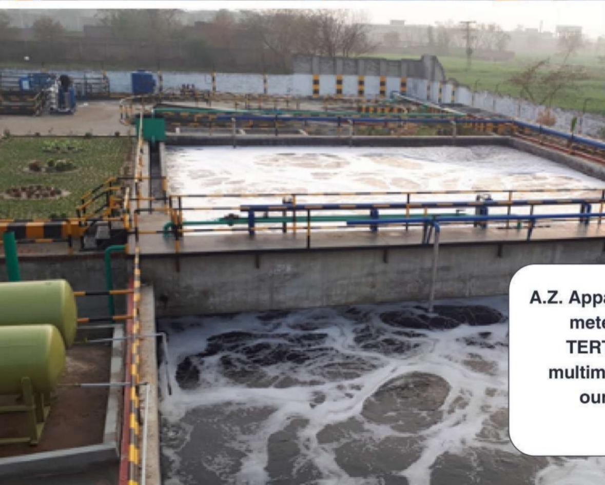
**A.Z. Apparel has installed biological treatment plant with capacity of 70 Cubic meters per hour. We are able to recycle 50% of waste water through TERTIARY TREATMENT which includes Ultra filtration, Disk filtration, multimedia filtration and Reverse Osmosis system. Thus, we are keeping ourselves in line with our social responsibilities by manufacturing sustainable, organic and Green to Wear products.**
